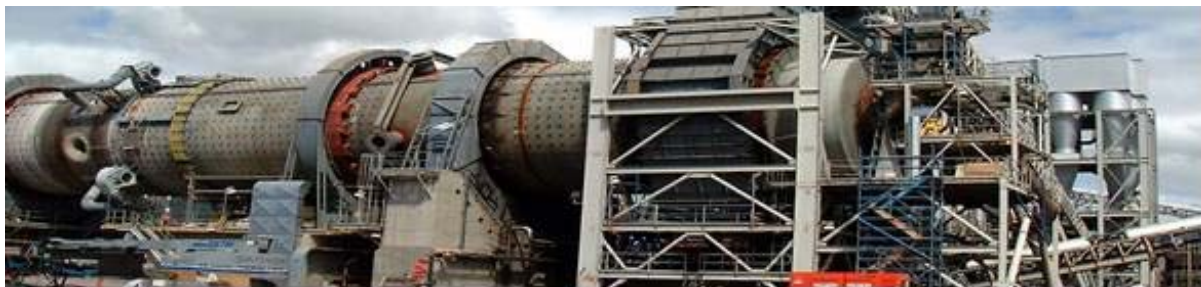
Figure 6: 210 ton per hour Alberta Taciuk Process (ATP) Retort (from AECOM, 2007)
